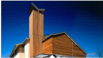
EVAPORATIVE COOLING TOWERS
