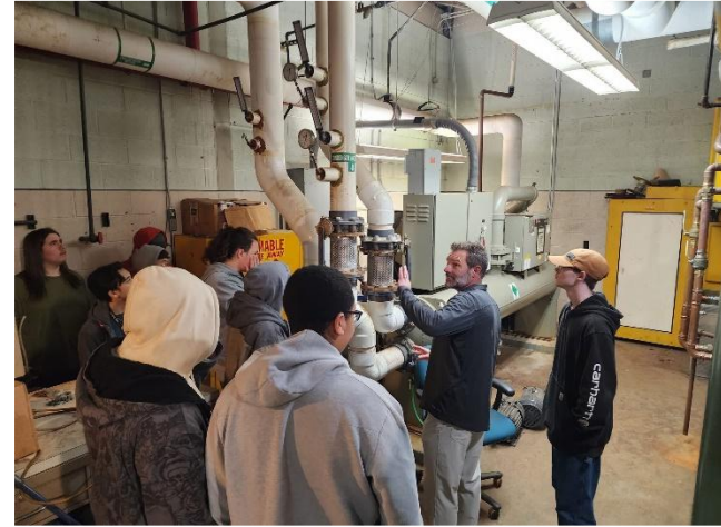
Energy Efficiency Job Shadow
